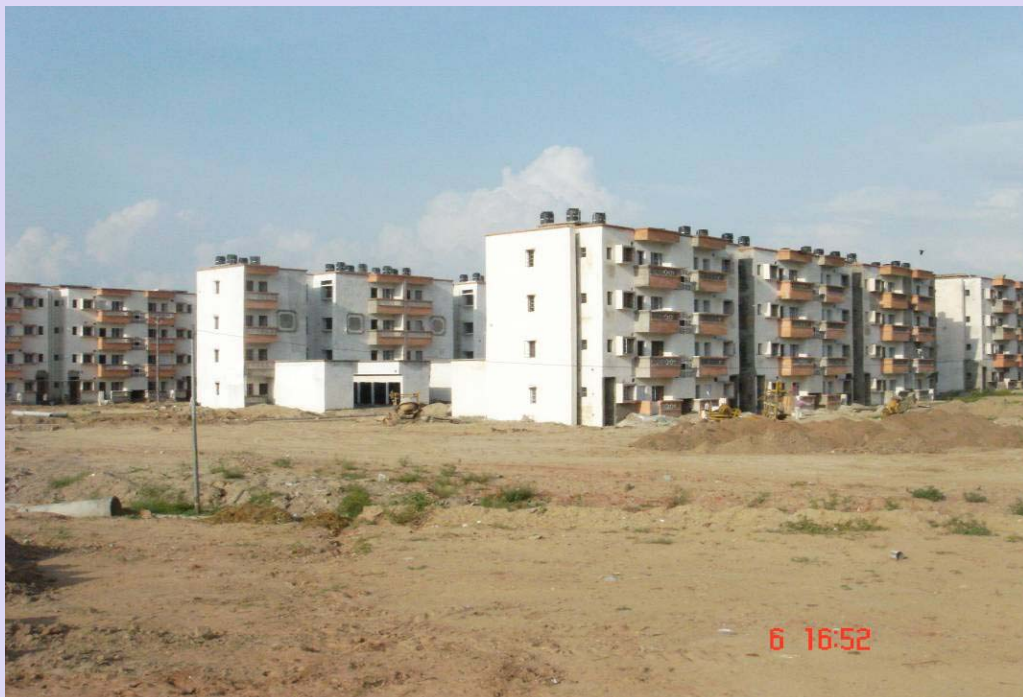
General view of buildings construction in Jaipur
