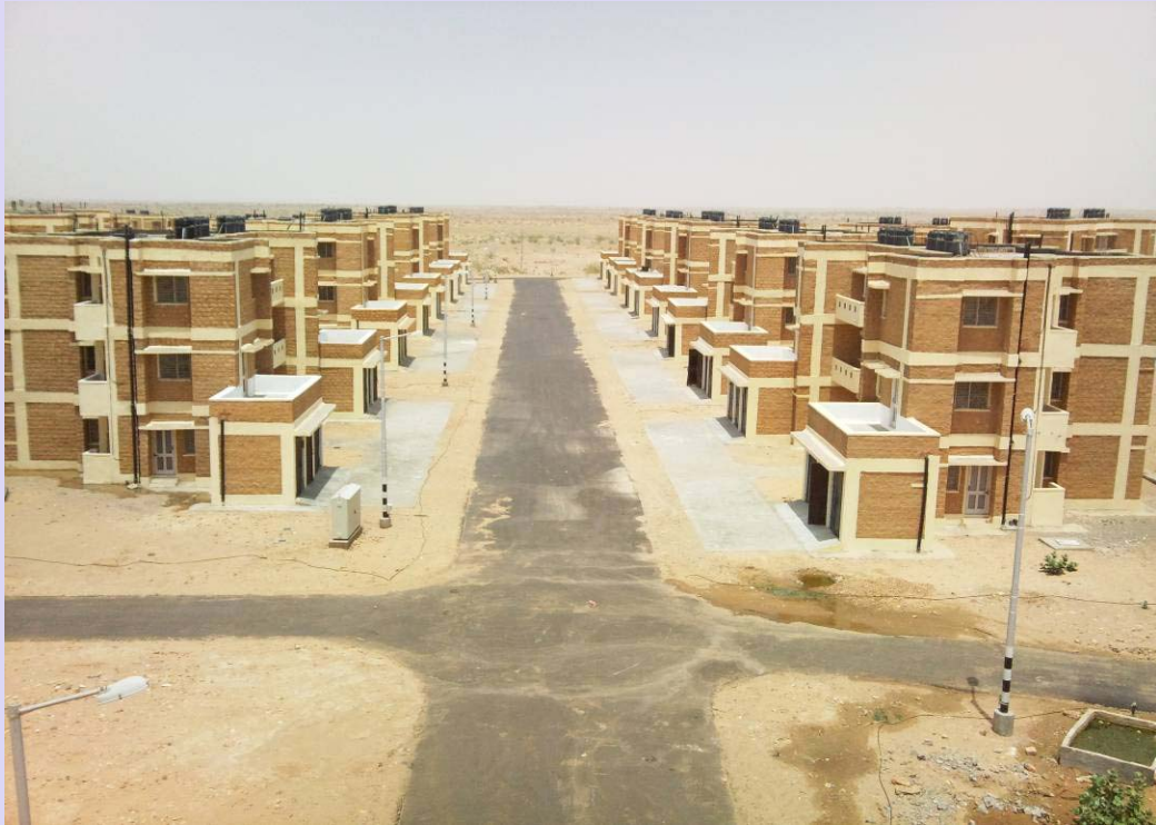
General view of the buildings constructed in Jaisalmer
