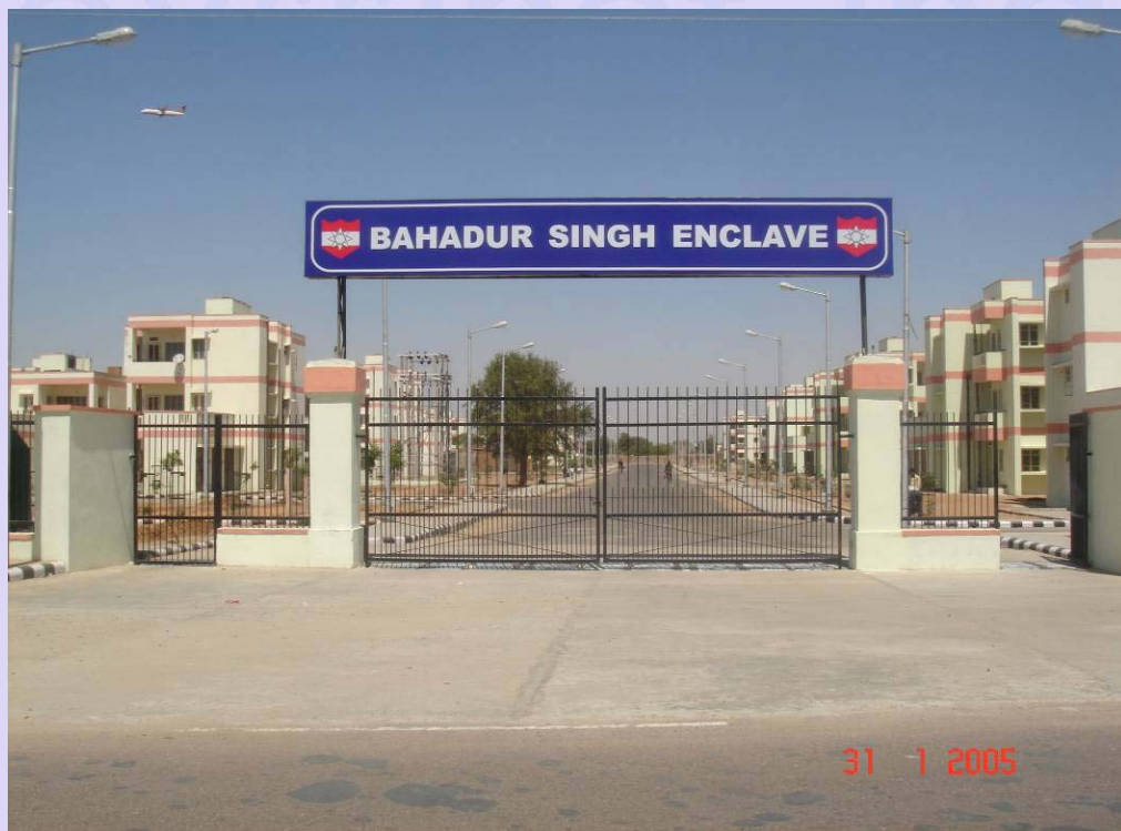
Entrance to the Enclave constructed in Shikargarh
