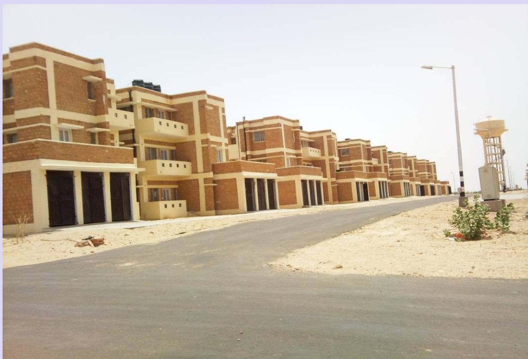
General view of the buildings constructed in Jaisalmer
