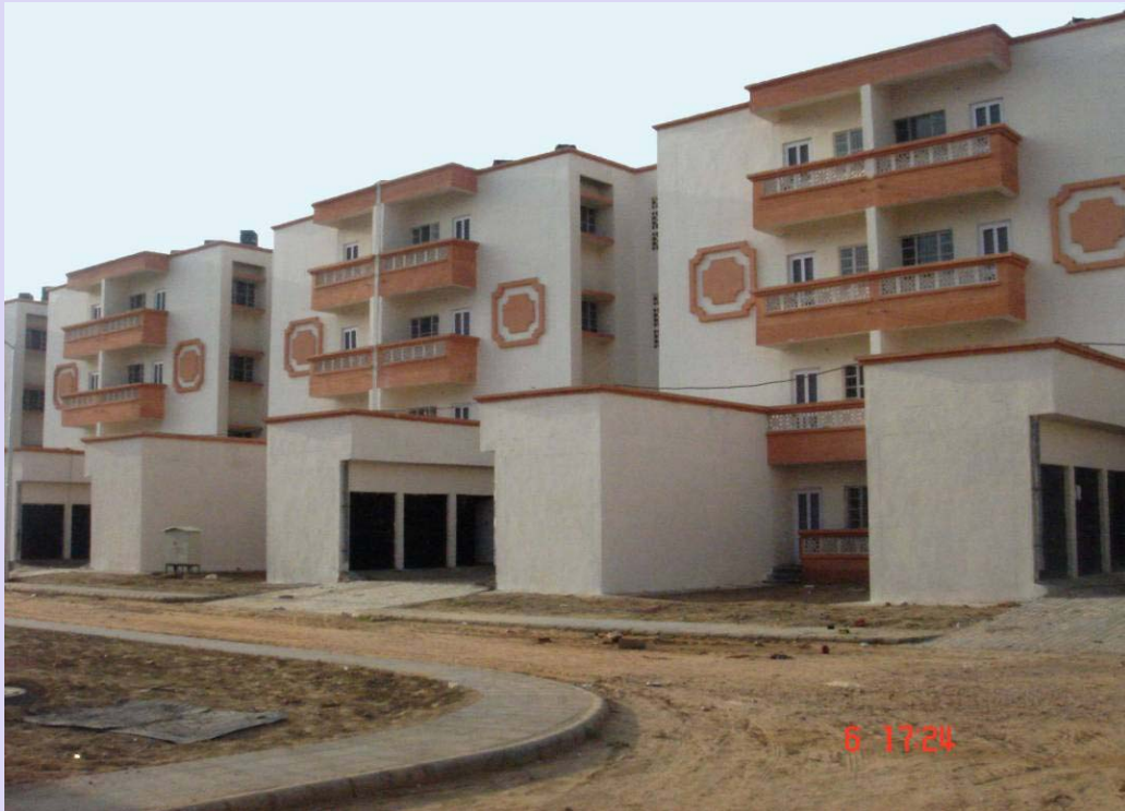
Close view of the buildings constructed in Jaipur
