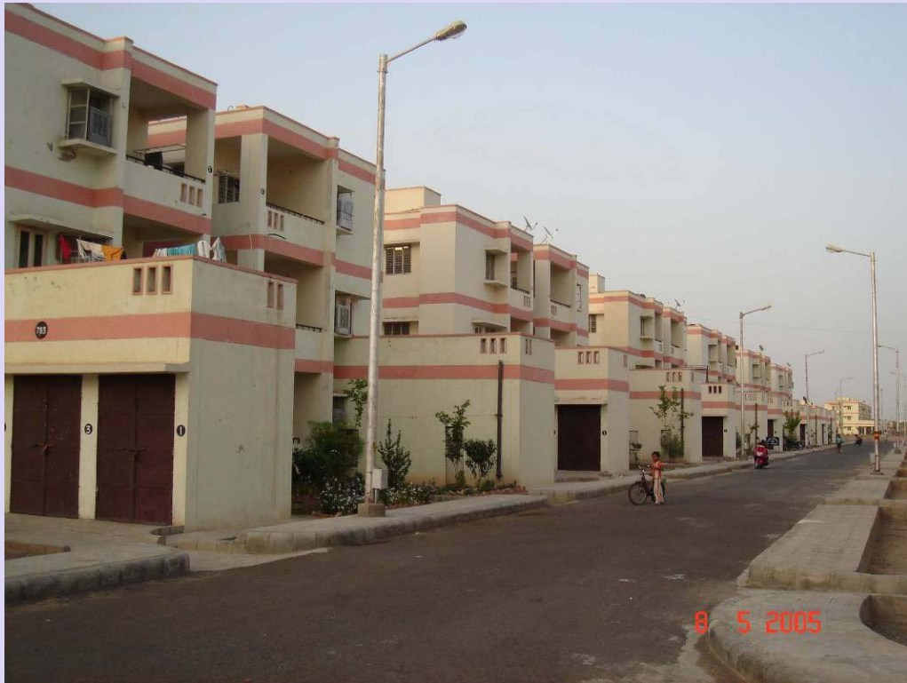
Buildings with access road in Shikargarh
