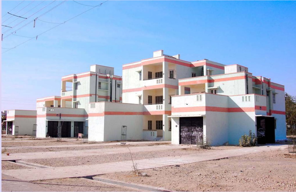
Typical view of building in Banar
