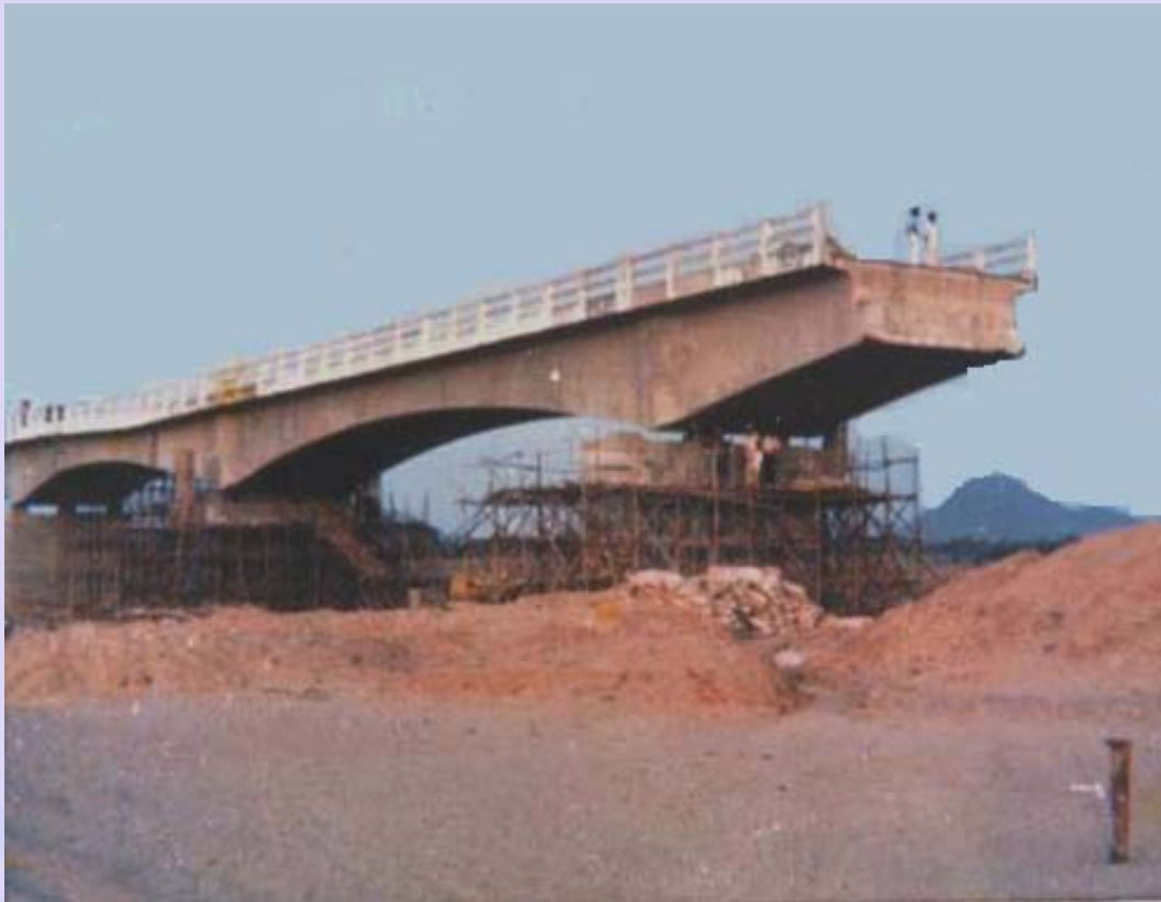
Vansadhara Bridge in Orissa State
