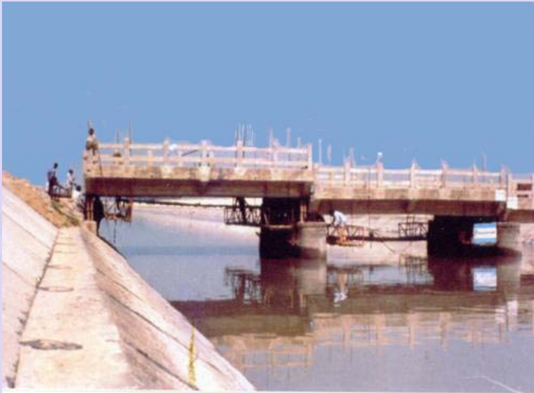
Sotlej Canal Bridge in Punjab
