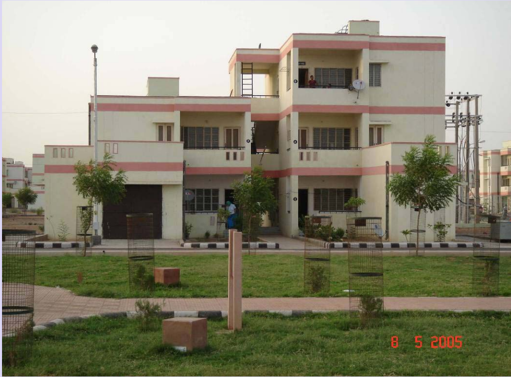
Typical view of building constructed in Shikargarh
